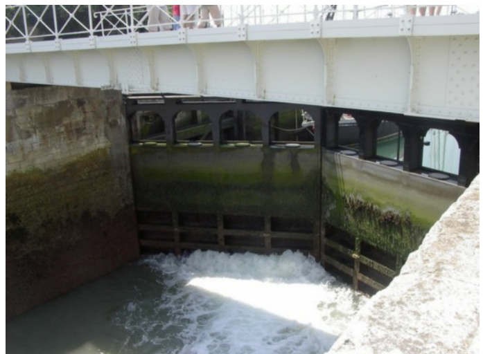
Below: The dock gate leaked for the whole tide cycle
